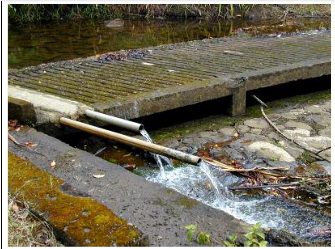
Hai'kū Ditch Intake, Honopou Stream, April 9, 2001 (two pipes drawing water from stream basin for family use); Flow estimated at 200,000 per 24 hour cycle (no rain in preceding day). (KPA Photo No. 1374)
