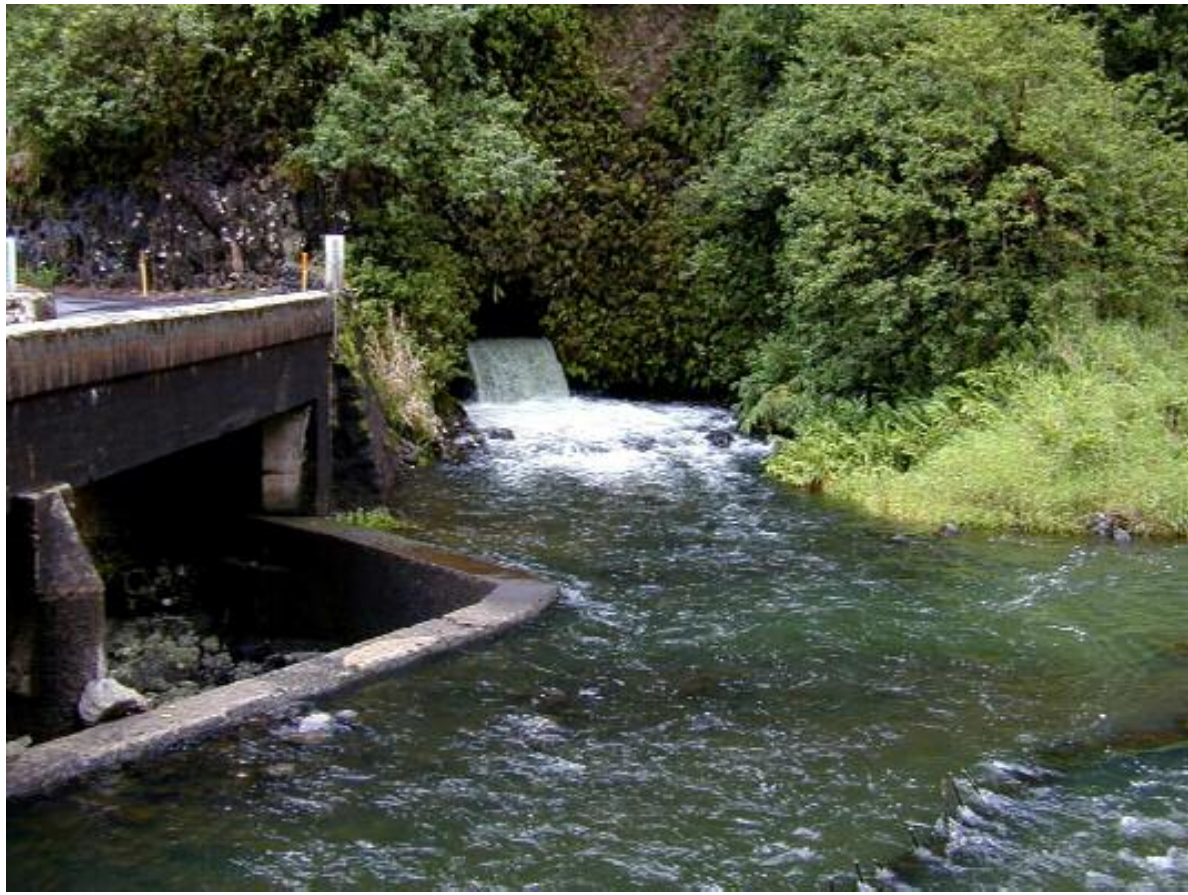
Kopili‘ula Stream – Ko‘olau Ditch Intake (KPA Photo No. 1469)
