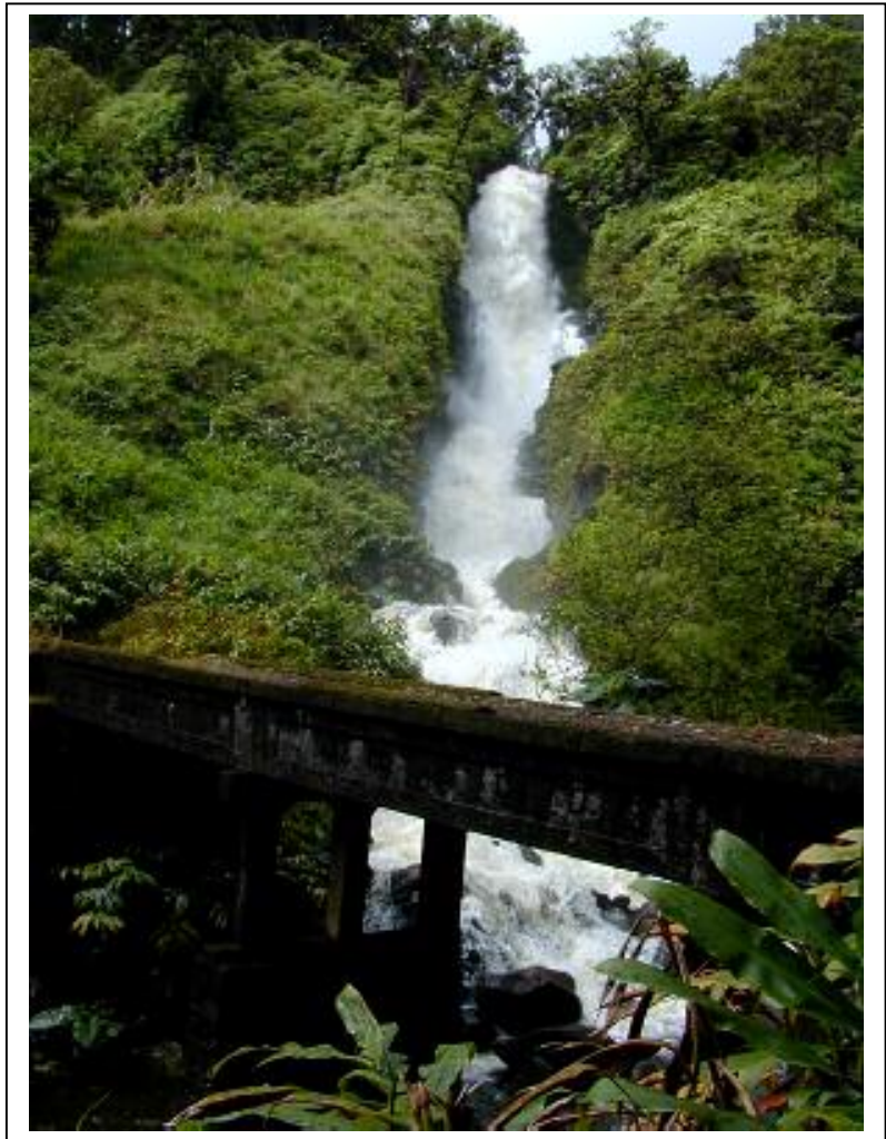
Spreckel's Ditch Overflow, Pu'ohākamoā Stream; EMI CO. Bridge (1925). (KPA Photo No. 1448)
