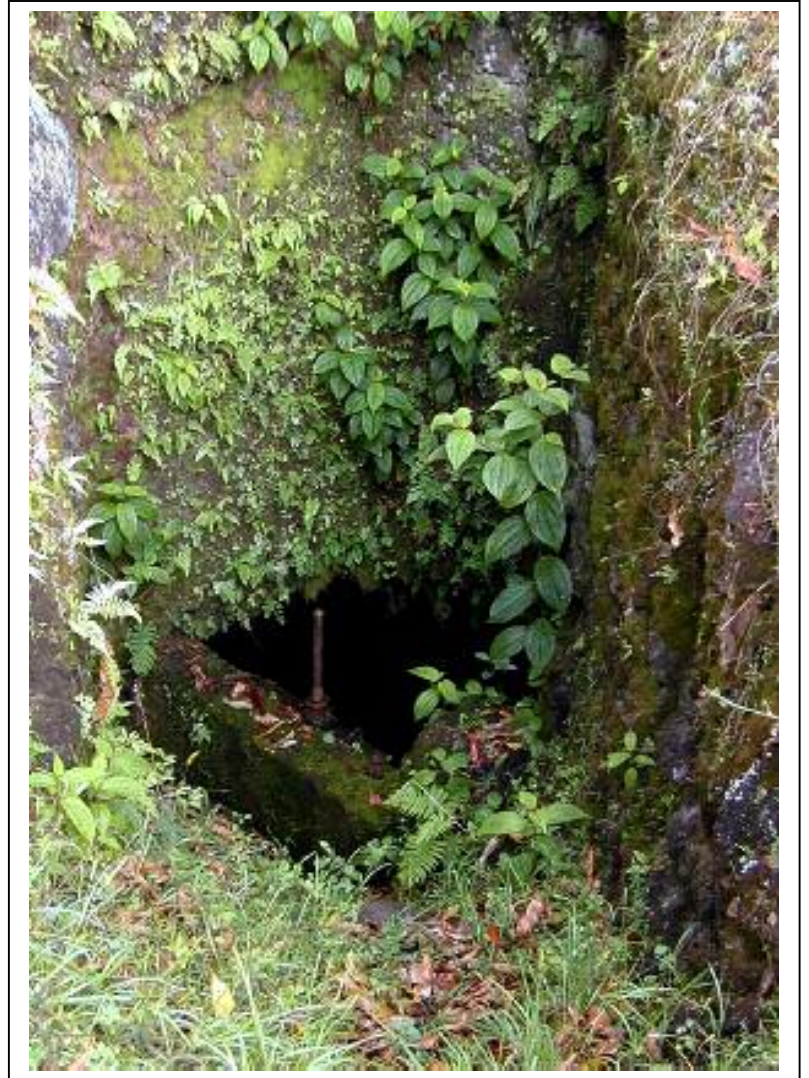
Old Water Gate for Honopou Residents – Ha'ikū Ditch (KPA Photo No. 1375)
